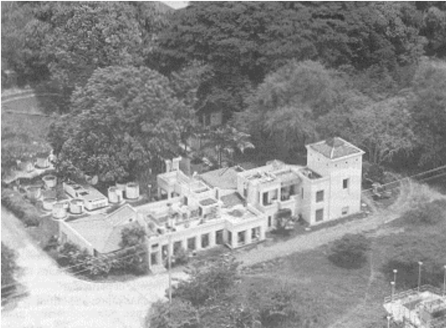
Figure 12: Comparing different MSF options in the research station in Puerto Mallerino, Cali, Colombia
