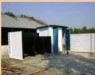
The biogas plant with inlets
