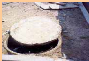
Covered disposal point of sludge
