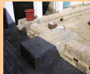
Sealed inlets facility to add cow dung
