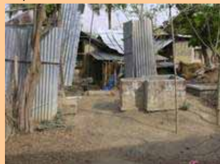
A community Biogas plant (human excreta based)
