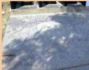
The desenter of Biogas plant
