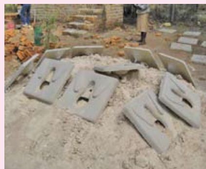
Concrete urine diverting EcoSan squatting pan made by the participants
