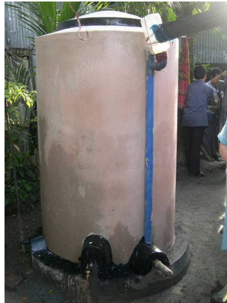
Fig. 2 Innovative RWH tank
