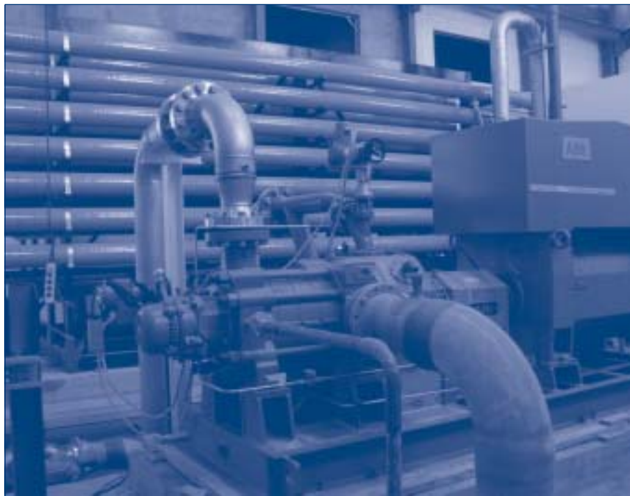
Fig. 18.11. Reverse osmosis (RO) racks and pump turbine system in La Aldea, Gran Canaria (capacity: 5000 m 3 /day; commissioned in 2001) (photograph by Jose M. Veza)
